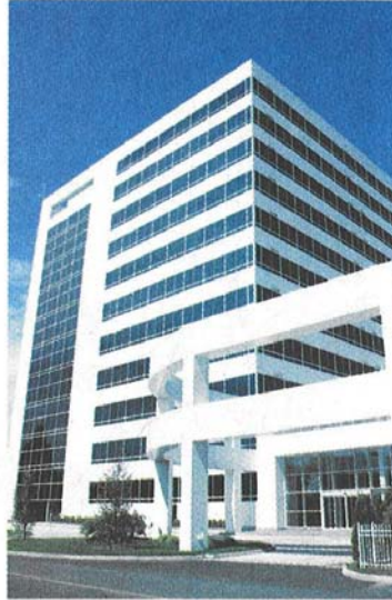
Hutchinson Metro Center.
